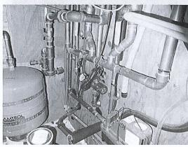
The domestic hot water is provided by the home heating plant. The temper valve installed to ensure that the water temperature is constant and uniform to the plumbing fixtures is accessible below the boiler (grey).
