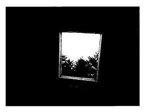
The bedroom skylight was stuck shut. I put a little force trying to open the skylight but was afraid I was going to cause damage to the skylight components. The skylight should operate for ventilation.
