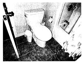
The toilet in the Jack and Jill bathroom on the 2<sup>nd</sup> floor is not properly secured to the floor. There was no water at the base of the toilet or leaks in the ceiling below the toilet, but the toilet should be secure.
