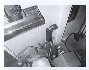
The water main shut off valve is located just above the floor to the left of the door in the utility closet. The interior finished sheet rock wall in the closet impedes on the operation of the water main shut off valve. The sheet rock should be cut away from the valve handle so the valve opens and closes unobstructed.
