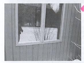
The bottom rails of the 1<sup>st</sup> floor bedroom windows at the front of the home are not properly sealed. The gasket at one of the windows is exposed.
