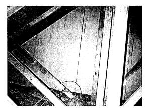
Sealing the sheet rock seams at the thermal wall in the attic with fire rated joint tape is recommended to slow an attic sourced fire from igniting the wood gable end structure.
