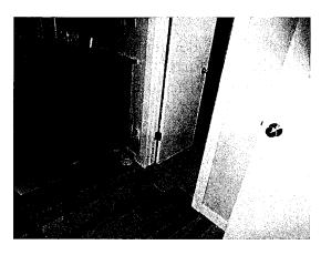
Subtle settlement was noted in the bedroom floor at the Jack and Jill bathroom doors. No cracks were noted in the interior finishes to indicate that the settlement was active or concerning. The settlement in the floor does represent a minor subfloor structure deficiency.
