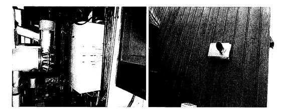
A 1-year-old split air-conditioner is installed in the enclosure at the rear of the home. Air handlers are installed on the interior walls to distribute the conditioned air in the winter and summer throughout the home.
