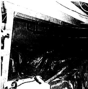
Photo 81-2 Vapor barrier is present on some of the crawlspace areas.
