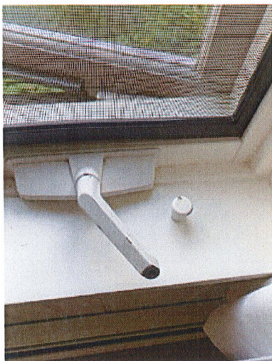
Photo 29-5 The window crank mechanism handle is in need of repair. Recommend repairs as needed by a qualified contractor.
