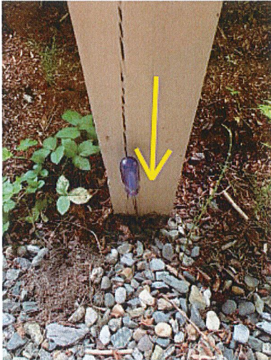
Photo 24-3 Deck support posts are below grade and have wood to earth contact, subject to eventual decay. No visible decay noted the day of inspection. Consider improving by installing proper concrete footings with wooden supports above grade (avoiding earth contact) by a qualified contractor.
