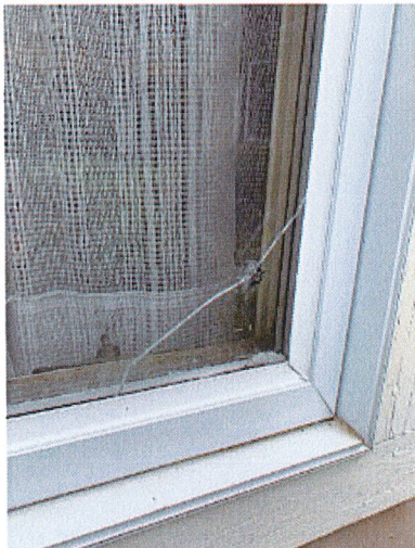
Photo 29-1 Broken glass in outer pane of garage window.
