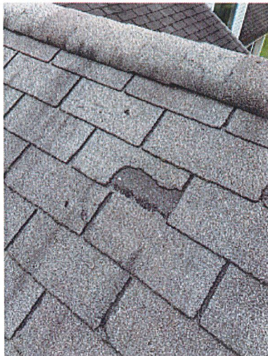
Photo 48-3 Deteriorated shingles with exposed nails. Potential for leaks.
