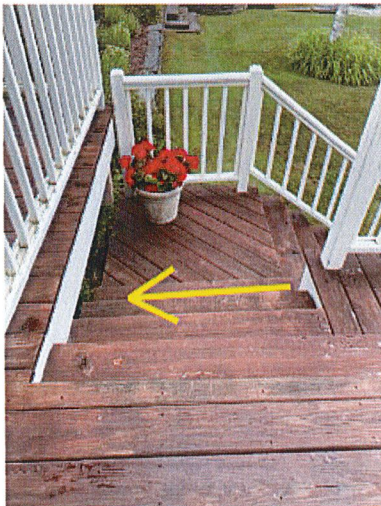
Photo 33-1 Tipped stairs may possibly be due to the rotten deck vertical support below.
