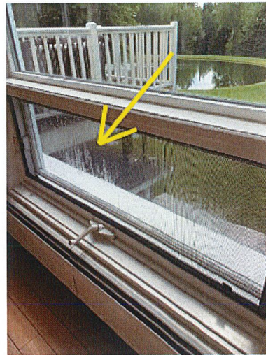
Photo 29-4 Seals between double-pane glass in one or more windows appear to have failed based on condensation or stains between the panes of glass. Recommend review and repairs or replacement as needed by a qualified contractor.
