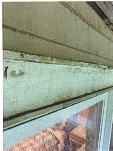
Photo 29-6 Basement bedroom window trim decay under deck.
