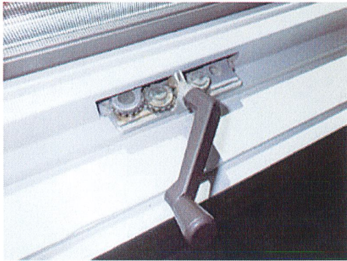
Photo 29-9 Casement window crank is missing its cover and presents a pinch hazard. Recommend installing cover where missing. This is the basement window to the left of the slider.
