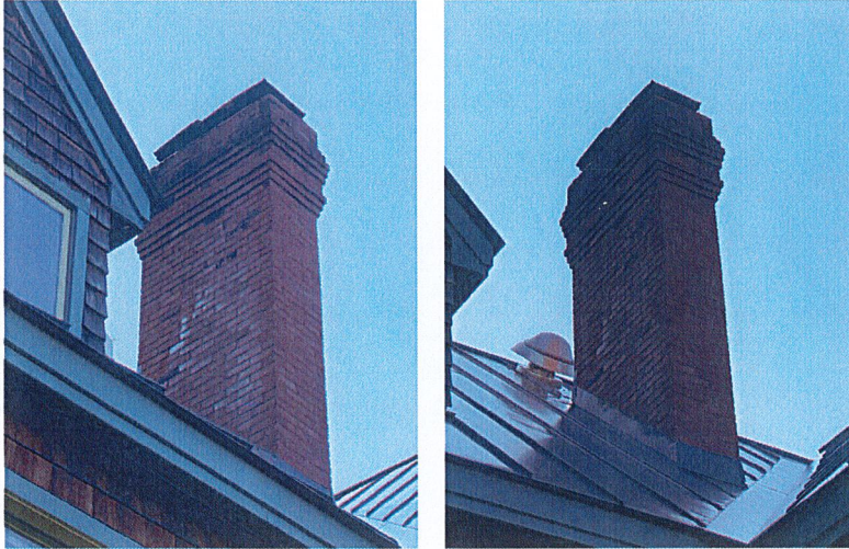
Three Flue Masonry Chimney
