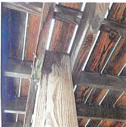
Photo 21-6 Connection is by lag bolts, not through bolting, monitor bolt at a minimum consider through bolting, deck
