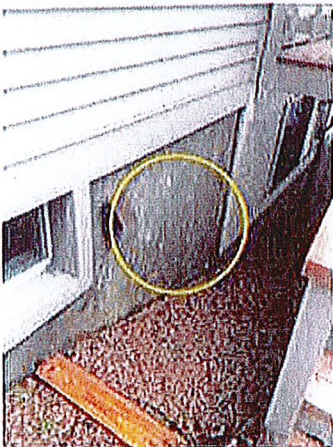
Photo 28-1 South side of home. Recommend repairs to parge coat covering the insulation.
