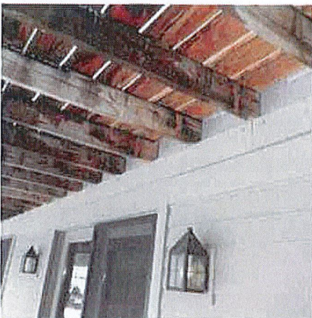
Photo 21-5 Deck joists are sitting on top of the ledger board with no bracing / joist hangers to prevent rotation of the
