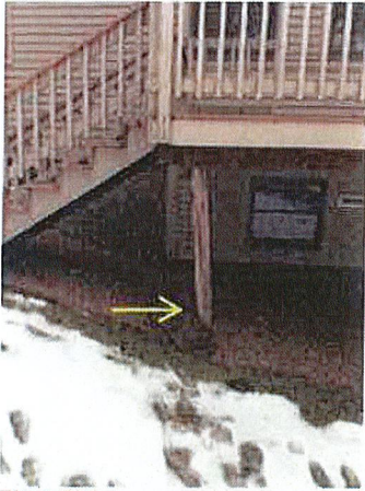
Photo 21-1 This vertical support is out of plumb and has been shimmed at its base. Recommend repairs as needed.
