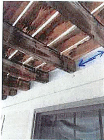
Photo 21-2 Recommend installing blocking between joists to prevent twisting. Ledger board has been bolted, flashing detail was noted. Only 2x6" joists used.
