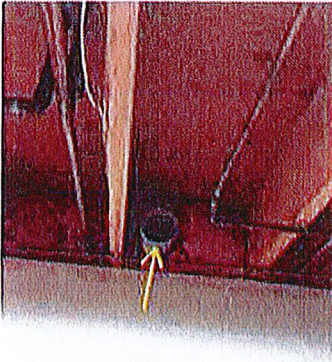
Photo 90-1 Basement bathroom fan termination.
