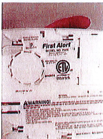
Photo 93-1 Battery operated photoelectric smoke detector located in the basement. It is not a 10-year lithium battery. Replace battery annually.
