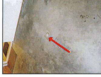
Garage floor drain
